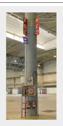
Note that the fire extinguisher equipment and sign need to remain accessible and visible at all times. These columns include a switchboard with 12 schuko type sockets of 10A to be used during build-up only.
